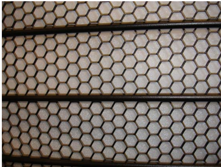
Figure 3: 80% Open Perforation on Front & Rear Doors
